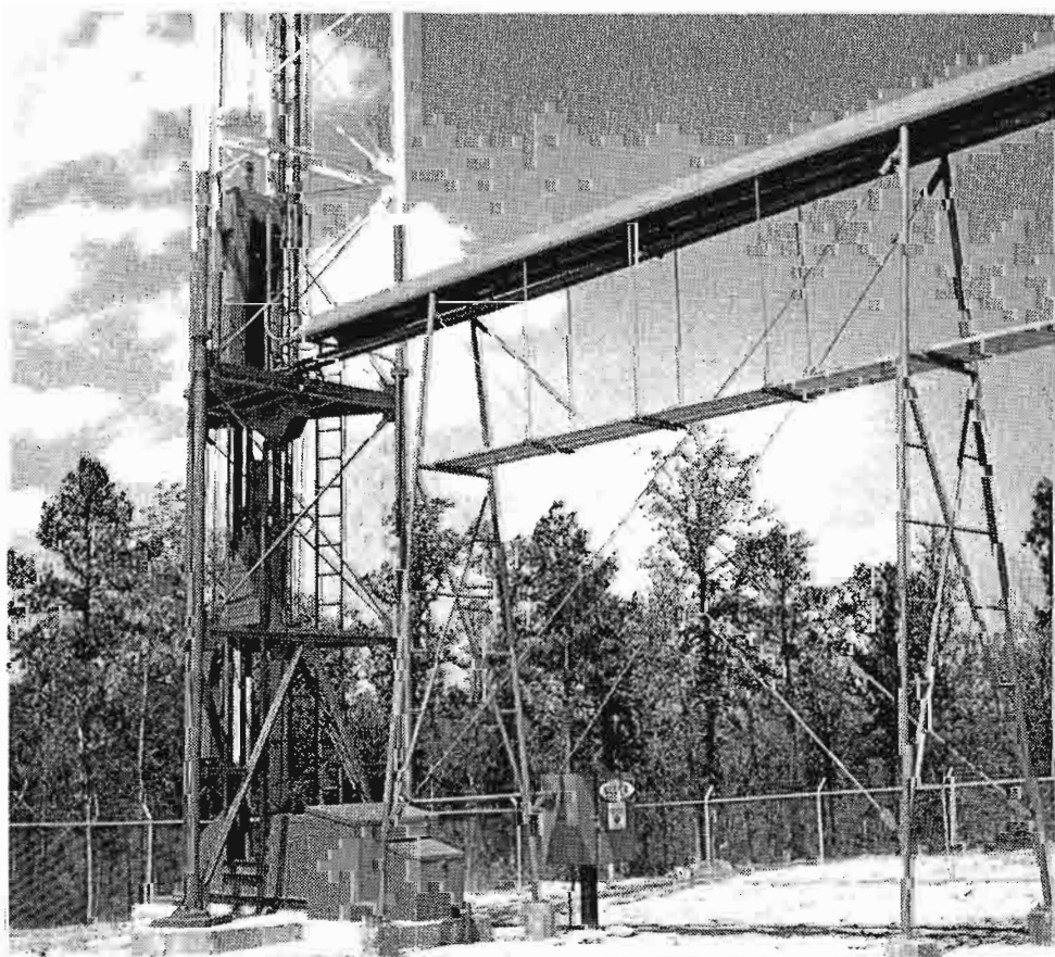
FIG. 6. Part of 80-ft run of transmission line running from tower to building. Inverted V-type steel cover plate protects line from falling ice.
